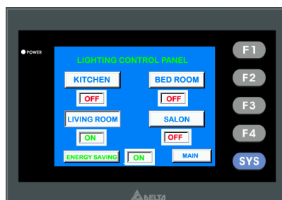
Figure 10 Lighting control panel
